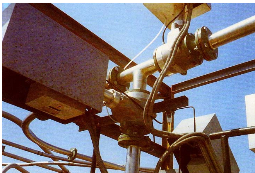
▶ Inlatable gasket slide valves type TSV-80 installed in pipelines operating with Nitrogen under positive pressure in a plant for producing Nylon 6.6 POY.
