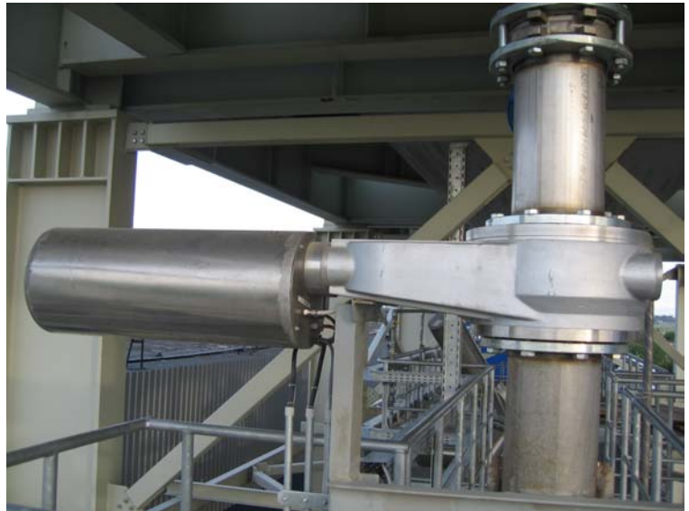
▲ MAB automatic slide valves type TSV-250 for installation with winterization, special execution for low ambient temperatures -40^{\circ}\text{C} .
