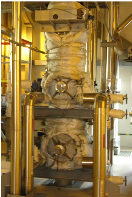
MAB high temperature rotary valves for PET chips at 210°C in SSP plant. Flow rate 18 t/hr – 500 t/day.
